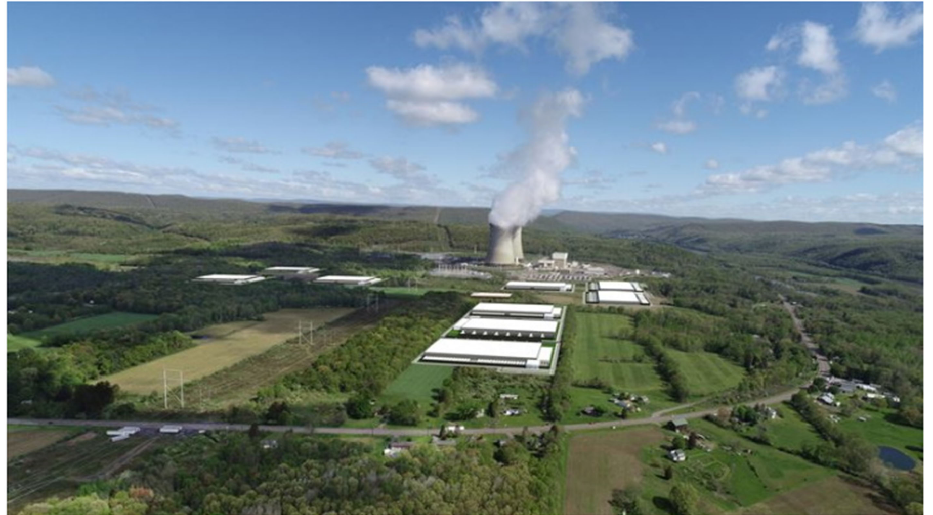
A rendering from 2021 of the data centre campus next to the Susquehanna power plant (Image: Linxon)
